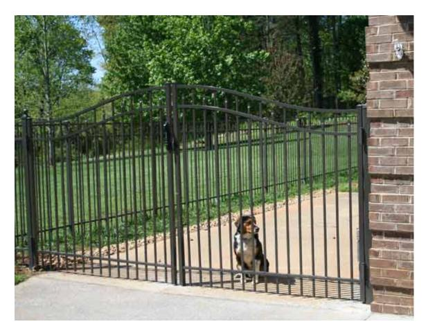
This is a double panel gate for vehicle access, boat, trailers, and large equipment. We like to set drop rods on BOTH gate panels for extra stability and security along with the other gate hardware. The double gate above is a decorative aluminum estate gate with gently sloping curves.
